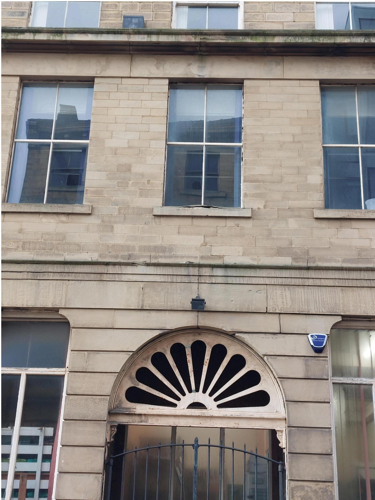
17-21 Chapel Street, East Elevation - Fan light and delaminating Ashlar Stone cill, window on floor above
