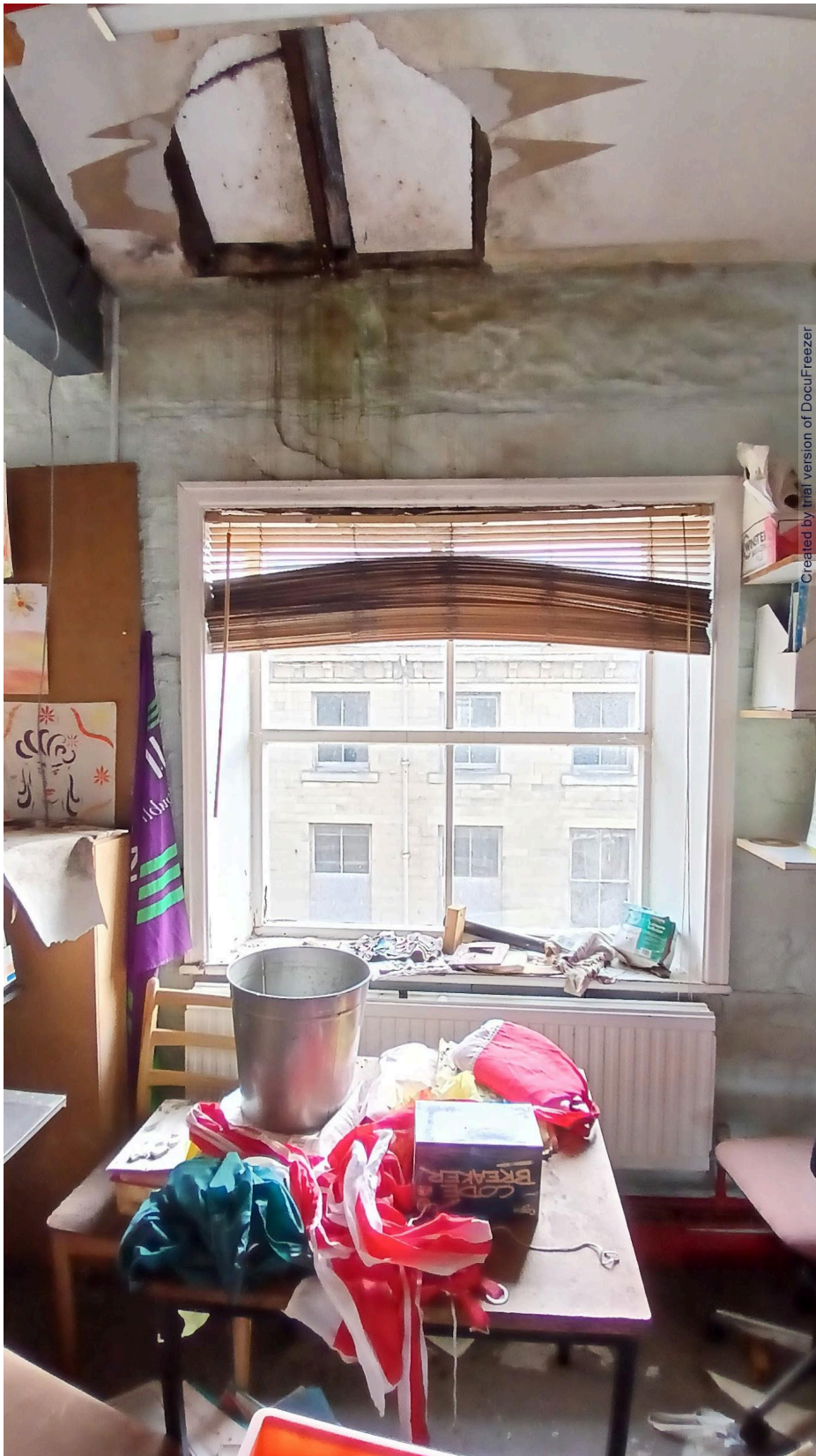
Water Ingress at Eaves - most likely caused by failure of the lead lined gutters directly above.
