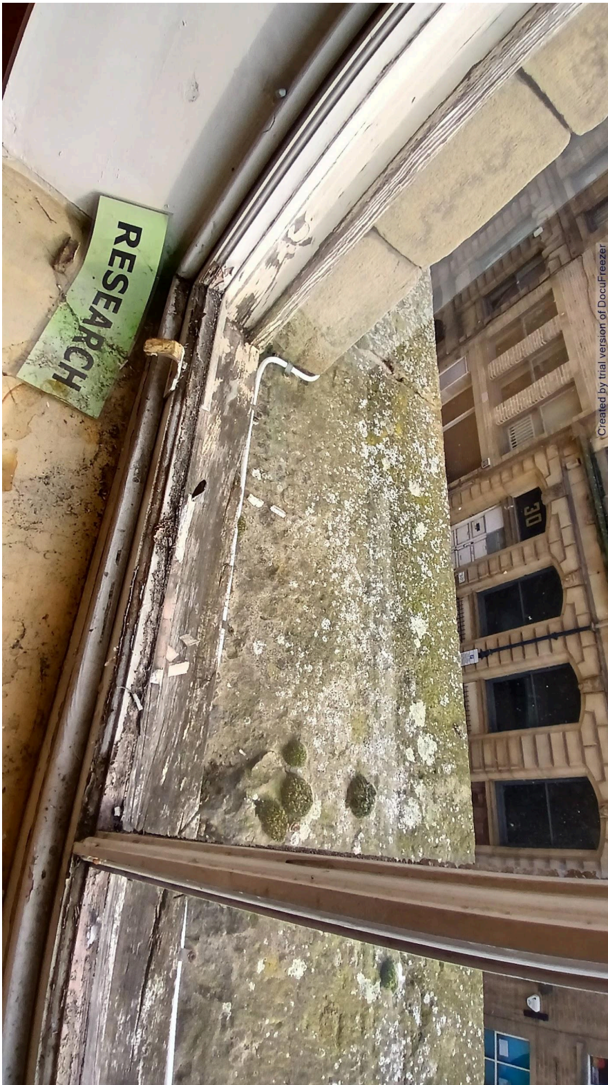
17-21 Chapel Street - Timber Decay in window, Chapel Street (East) Elevation
