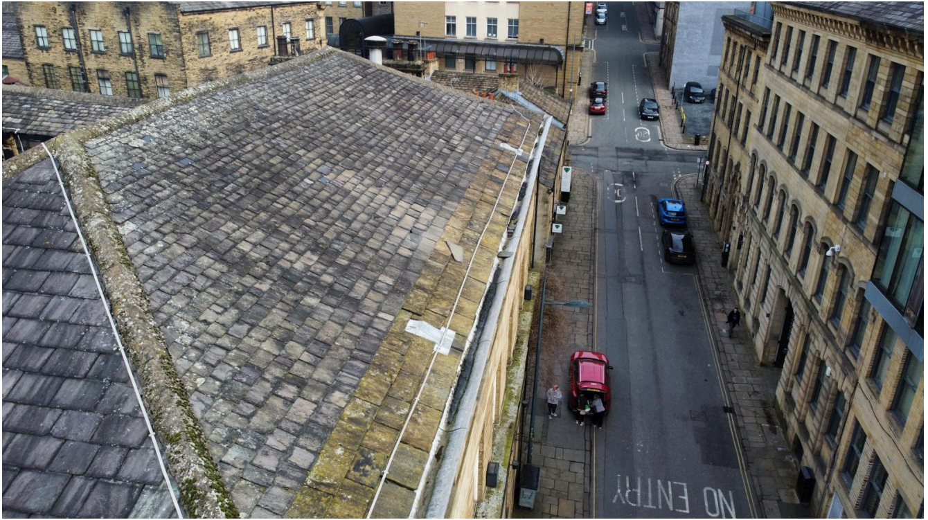
17-21 Chapel Street - Main Roof, (east) Chapel Street Elevation showing the lead-lined gutter, three courses of Westmorland Stone slates to eaves with traditionally laid diminishing courses of Welsh slate above.
