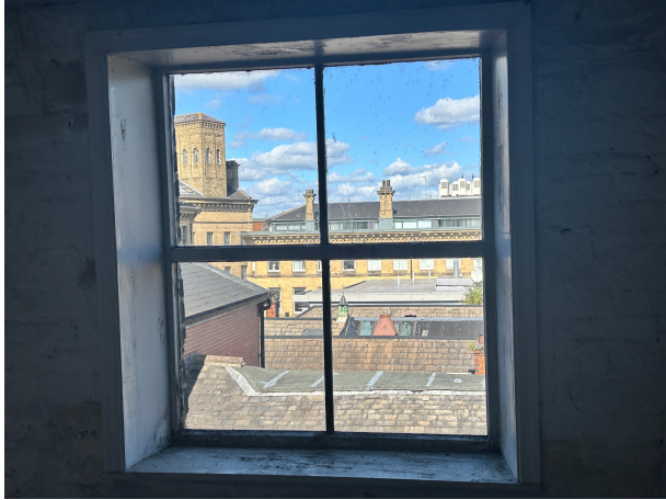
Figure 4 (above): Internal window (West facing)
