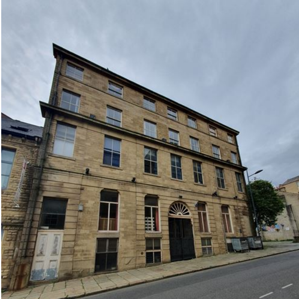
Figure 1: Front façade to Chapel Street, Bradford
